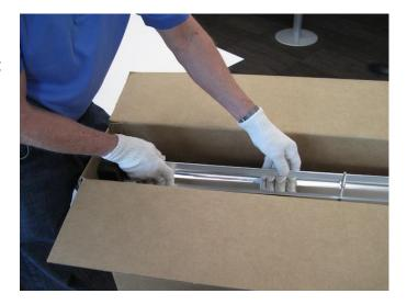
Note: DO NOT set the LightLouver unit down directly onto the floor, as this can cause damage to the "footer" components that cap the bottom end of each vertical support rod. If the LightLouver unit must be set down, place a piece of 1" X 4" packaging foam on the floor first, and then set the LightLouver unit on the foam.
