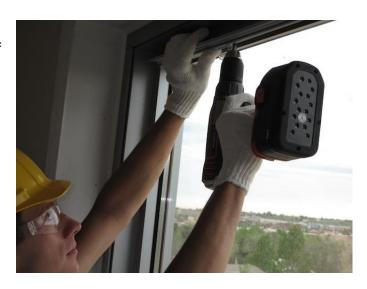
aluminum as it passes through, creating a cleanly tapped hole. Repeat process with two screws per support bracket, taking care to ensure that all brackets are aligned correctly with the front parallel to the glass. This will ensure that the valance is straight after installation.
