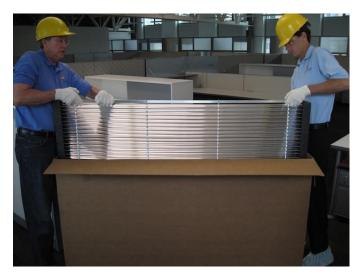
Two people, one on either end of the LightLouver unit, should gently grasp the bottom slat with one hand, and support the back of the top slat with the other hand. Both hands should be located as closely as possible to where the nearest vertical support rod runs through the slats.
