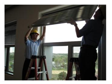
7. Ensure that the LightLouver unit is centered between the window mullions. If adjustment is
