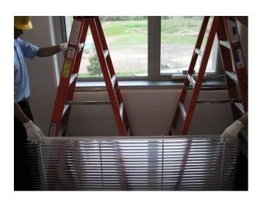
With the reflective surface of the slats (inside surface) facing up, and holding the LightLouver unit at a 45 degree angle with the top edge closest to the window and the bottom edge furthest, pass the horizontal aluminum header bar through the openings in the support brackets.
