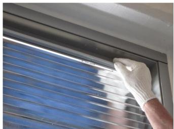
8. Perform a final inspection of the installed LightLouver unit before installing the next LightLouver unit. Remove any observable dust, fingerprints, or smudges on the reflective surfaces using the dusting and glass cleaning products provided with the product. All cleaning and maintenance MUST be performed in accordance with the LightLouver Maintenance Manual.
