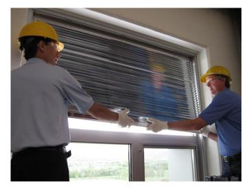
Pivot the valance into the "closed" position so that the header bar is no longer visible. The valance should lock into position on the support brackets with an audible click when fully closed.
