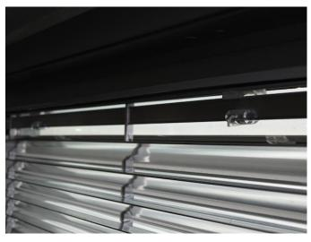
It may be necessary to gently and slightly "twist" the unit if it is no longer perfectly square due to shipping or installation movement. Likewise, if any unit twisting is apparent, it may be necessary to gently correct the twist so that the LightLouver unit is positioned flat in the window. If excessive twisting, racking, or warping is observed and cannot be readily corrected, please contact LightLouver LLC.
