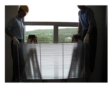
Continue to apply moderate pressure upwards and towards the glass, and carefully allow the bottom edge of the LightLouver unit horizontal support bar to pivot downward into the resting position in the support brackets. Once released, the LightLouver unit should hang vertically with all of the "footer" components contacting the glass.
