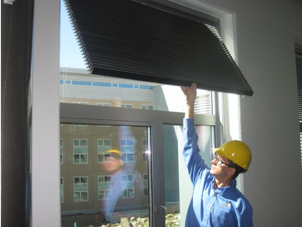
Figure 5: LightLouver unit being opened
