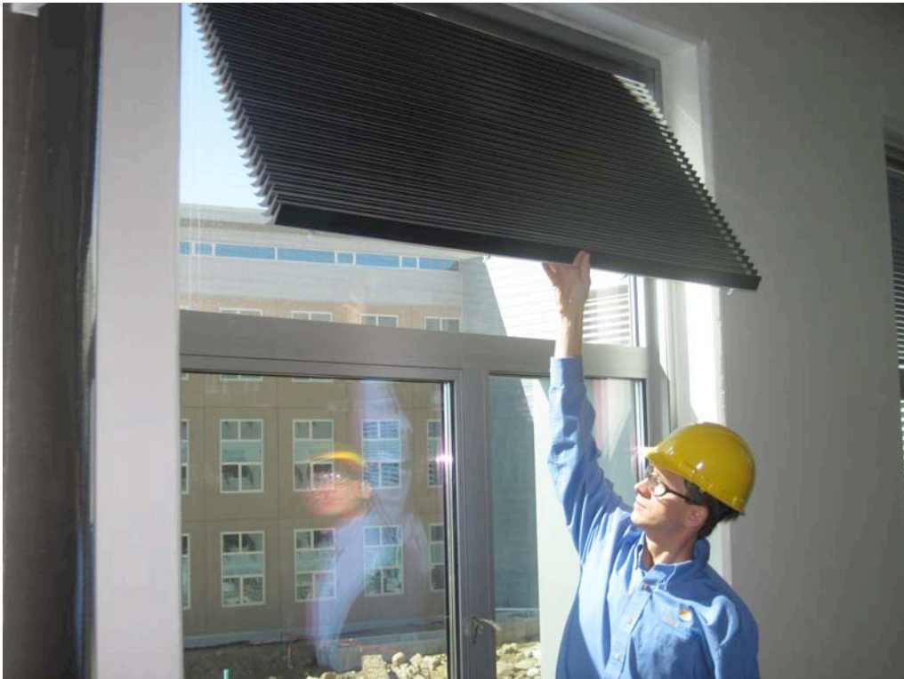
Figure 5: LightLouver unit being opened
