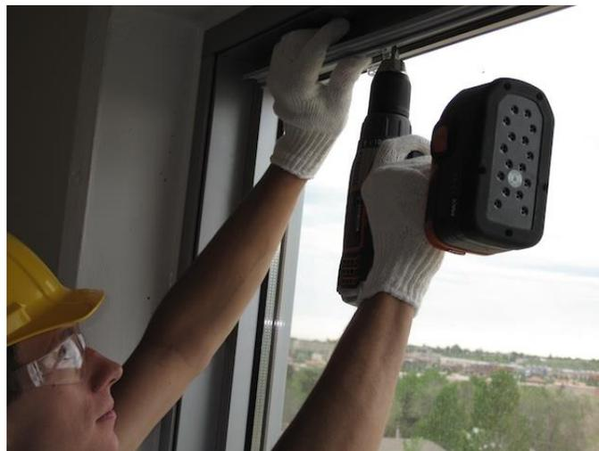
aluminum as it passes through, creating a cleanly tapped hole. Repeat process with two screws per support bracket, taking care to ensure that all brackets are aligned correctly with the front parallel to the glass. This will ensure that the valance is straight after installation.
