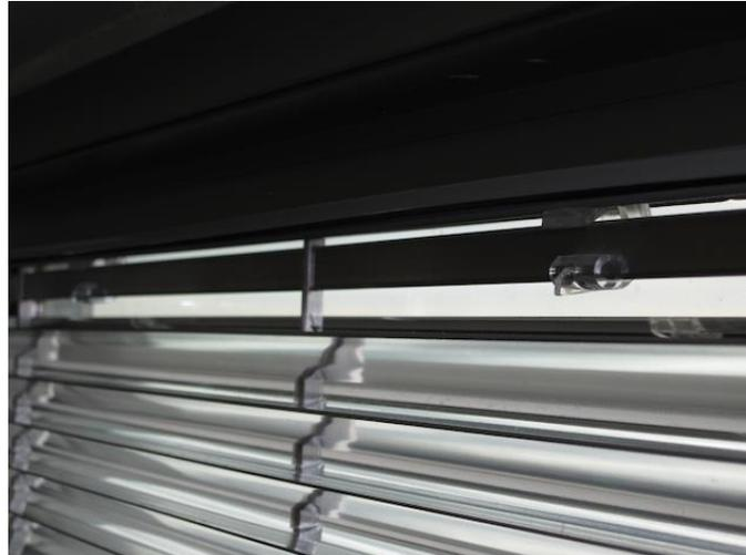
It may be necessary to gently and slightly “twist” the unit if it is no longer perfectly square due to shipping or installation movement. Likewise, if any unit twisting is apparent, it may be necessary to gently correct the twist so that the LightLouver unit is positioned flat in the window. If excessive twisting, racking, or warping is observed and cannot be readily corrected, please contact LightLouver LLC.
