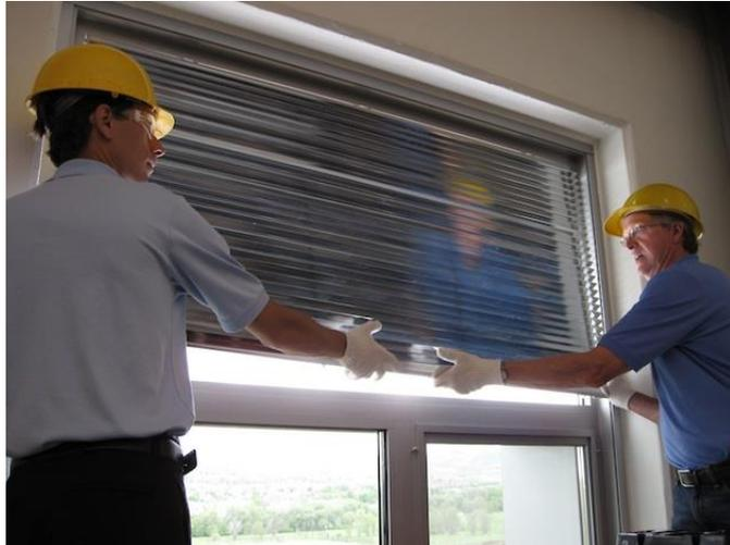
Pivot the valance into the “closed” position so that the header bar is no longer visible. The valance should lock into position on the support brackets with an audible click when fully closed.
