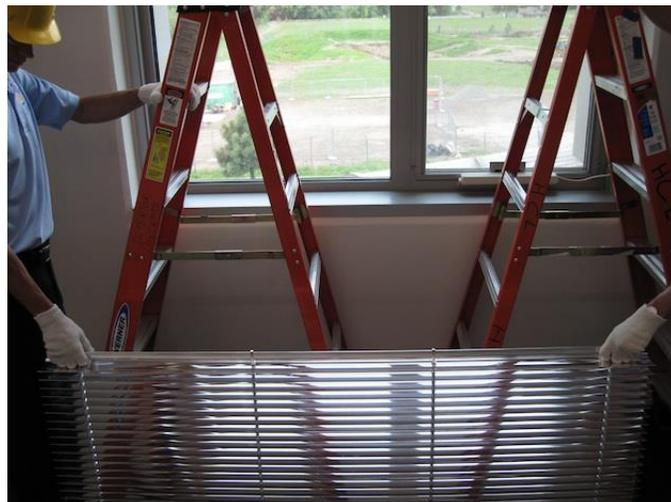
With the reflective surface of the slats ( inside surface ) facing up, and holding the LightLouver unit at a 45 degree angle with the top edge closest to the window and the bottom edge furthest, pass the horizontal aluminum header bar through the openings in the support brackets.
