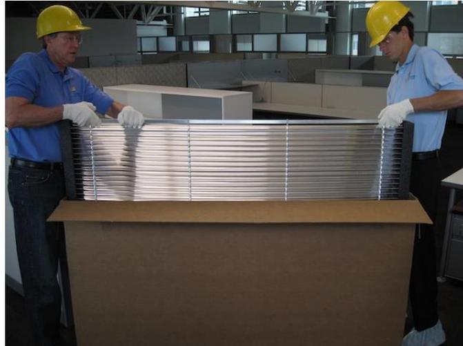
Two people, one on either end of the LightLouver unit, should gently grasp the bottom slat with one hand, and support the back of the top slat with the other hand. Both hands should be located as closely as possible to where the nearest vertical support rod runs through the slats.
