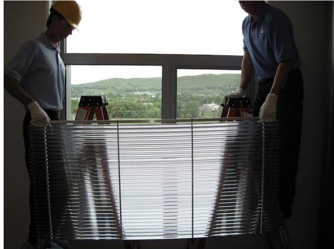
Continue to apply moderate pressure upwards and towards the glass, and carefully allow the bottom edge of the LightLouver unit horizontal support bar to pivot downward into the resting position in the support brackets. Once released, the LightLouver unit should hang vertically with all of the “footer” components contacting the glass.
